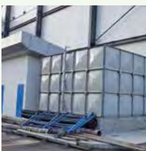
Our 1st rain water harvesting tank in Pulau Indah.
