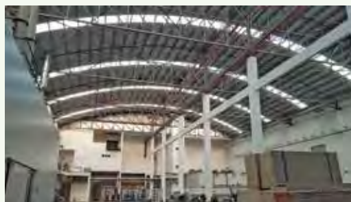
Natural lighting for main raw material storage area and production floor in Kawan's Pulau Indah facility.
